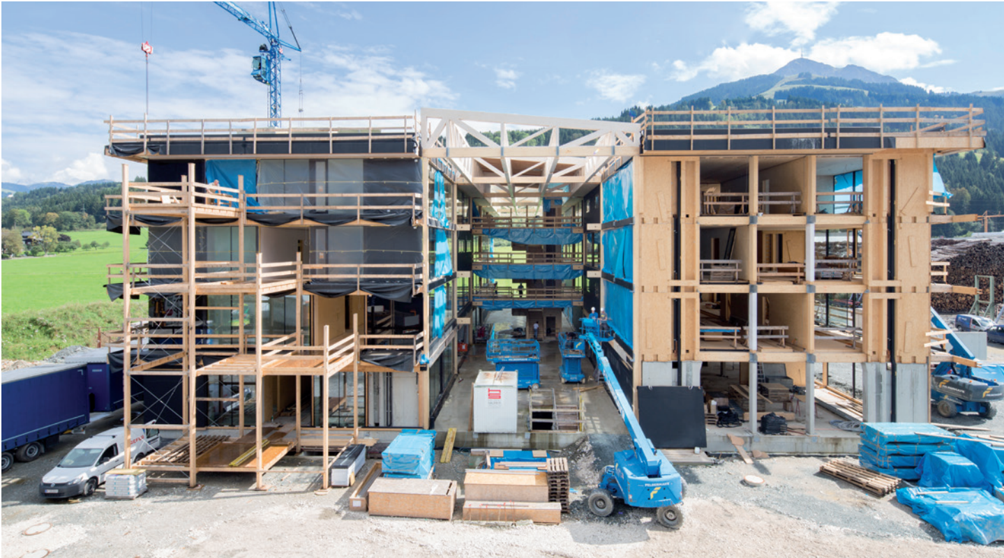
The construction phase - the building complex was erected in a year
